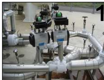
PHOTO 1: ball valves for cryogenic service (oxygen, nitrogen, liquefied natural gas) PHOTO 2: ball valves for oil and LPG PHOTO 3: ball valves with pneumatic actuator PHOTO 4: ball valves for gas purification
